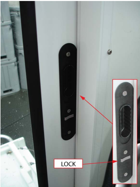
Photo 4. Port door interior latch
