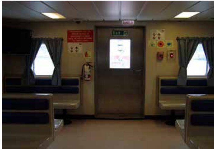
Photo 5. Aft exit of passenger lounge (lifejackets outside door on deck but no signage)
