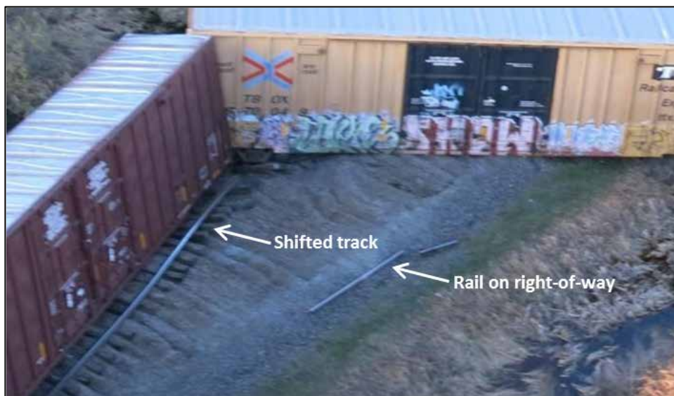
Photo 5. West end of the derailment site showing the shifted track and 2 pieces of rail on right-of-way (Source: Forest Helicopters Inc.)
