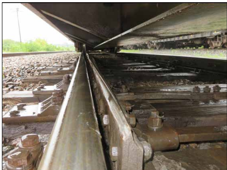
Photo 2. Left switch point (east)
