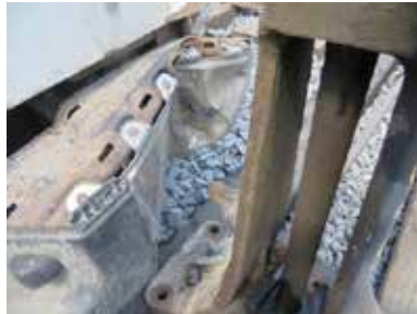
Photo 6. Damage to the pickup truck's bumper
