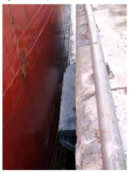
Figure 6. Illustration of spring lines caught under fender
