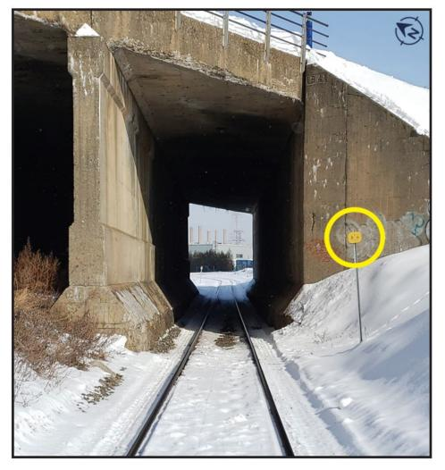
At the western end of track PD06, signal 410RC controls access to the Montreal Subdivision main track.
